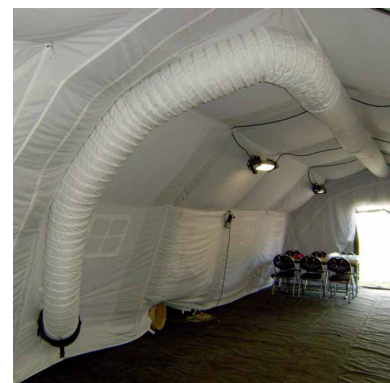
Air distribution plenums.
