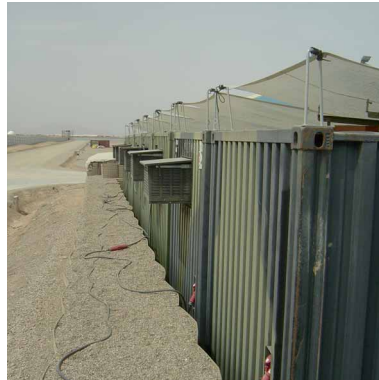
Container cooling with ACM 5.
